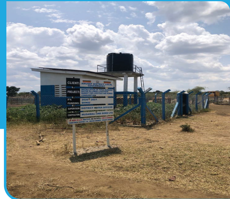
The piped water supply system at Loro livestock market which generates revenue that contributes to maintenance of the market.
