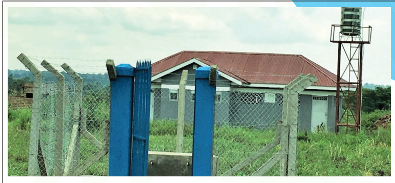
Fig 4: The Adibo Public water borne Sanitation Facility
